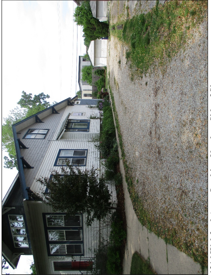
1316 Webford Ave – Looking North at Side of Site
