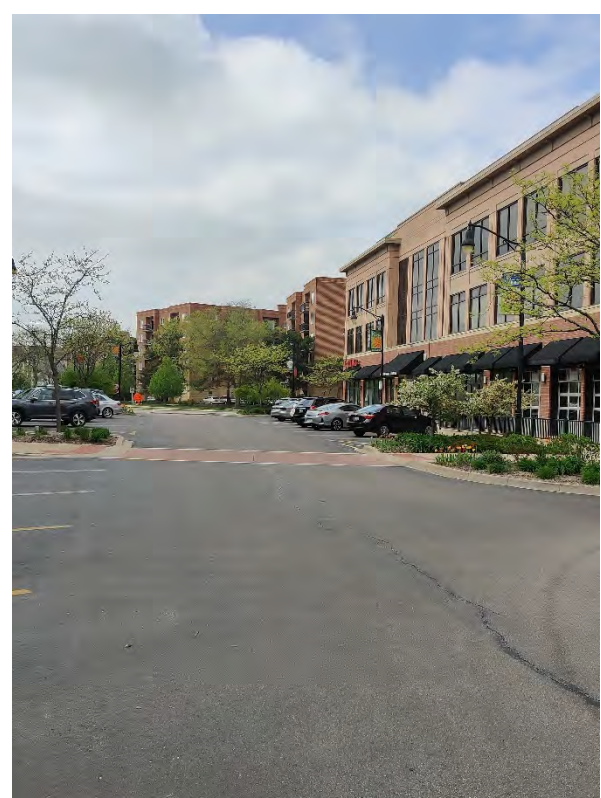
Metropolitan Square – Facing West
