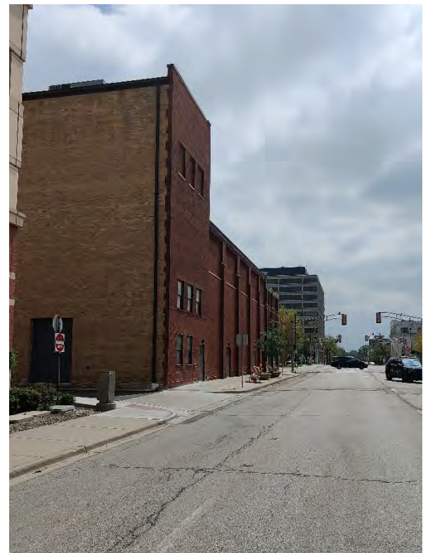
1470-1476 Miner St – Facing Southeast
