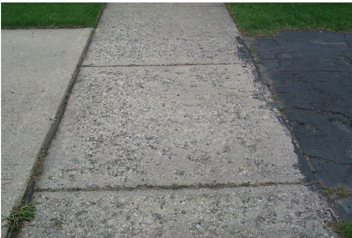
Figure 5 – Pitted Sidewalk
