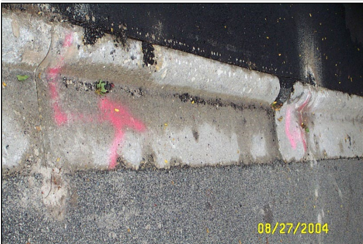
Figures 11 & 12 - Deteriorated Curb, Asphalt Apron (Before and After)
