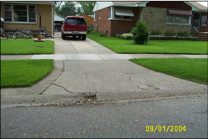
Figures 13 & 14 - Deteriorated Curb and Cracked Apron if it is creating drainage issues in the pavement
