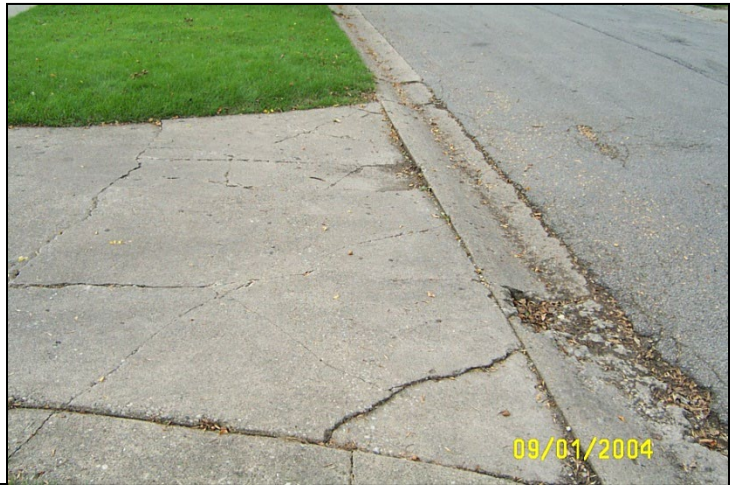
Figures 13 & 14 - Deteriorated Curb and Cracked Apron if it is creating drainage issues in the pavement
