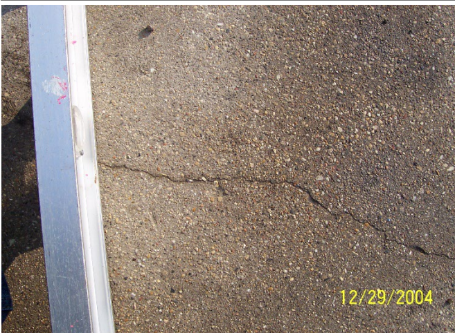
Figures 7 & 8 – Hairline Crack in Sidewalk
