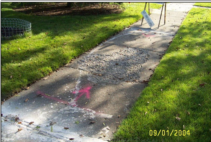
Figure 3 – Deteriorated Sidewalk
