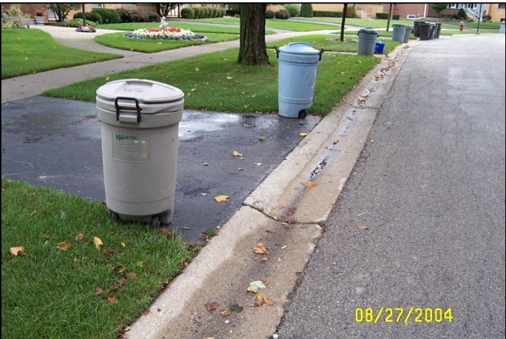
Figures 15 & 16 – Rolled Curb in Good Condition
