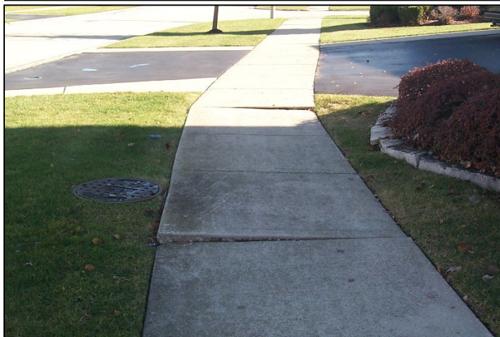
Figure 4 – Tilting Sidewalk
