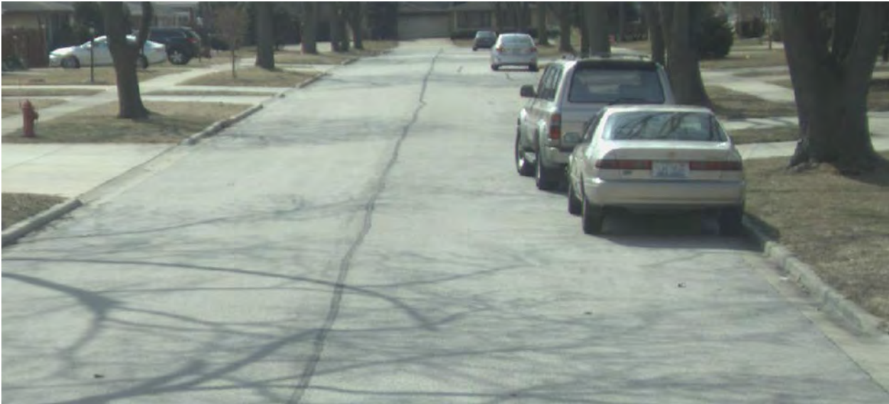
Figure 3-7: Orchard Street Section 10, PCI 91 (Good)
