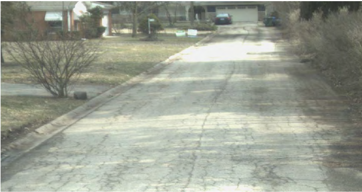
Figure 3-16: Hawthorne Terr Section 00, PCI 14 (Serious)
