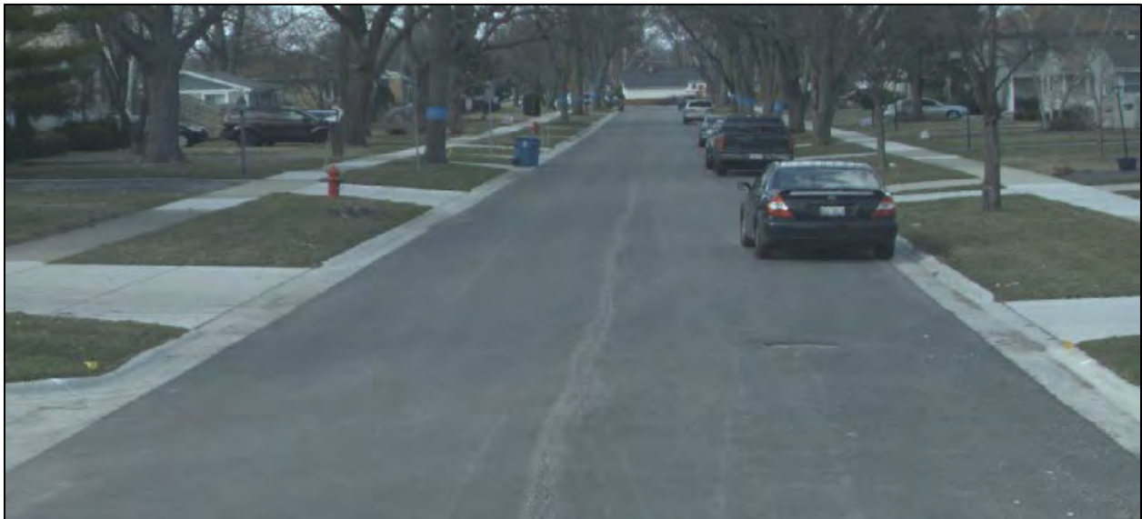
Figure 3-6: Cedar Street Section 05, PCI 100 (Good)
