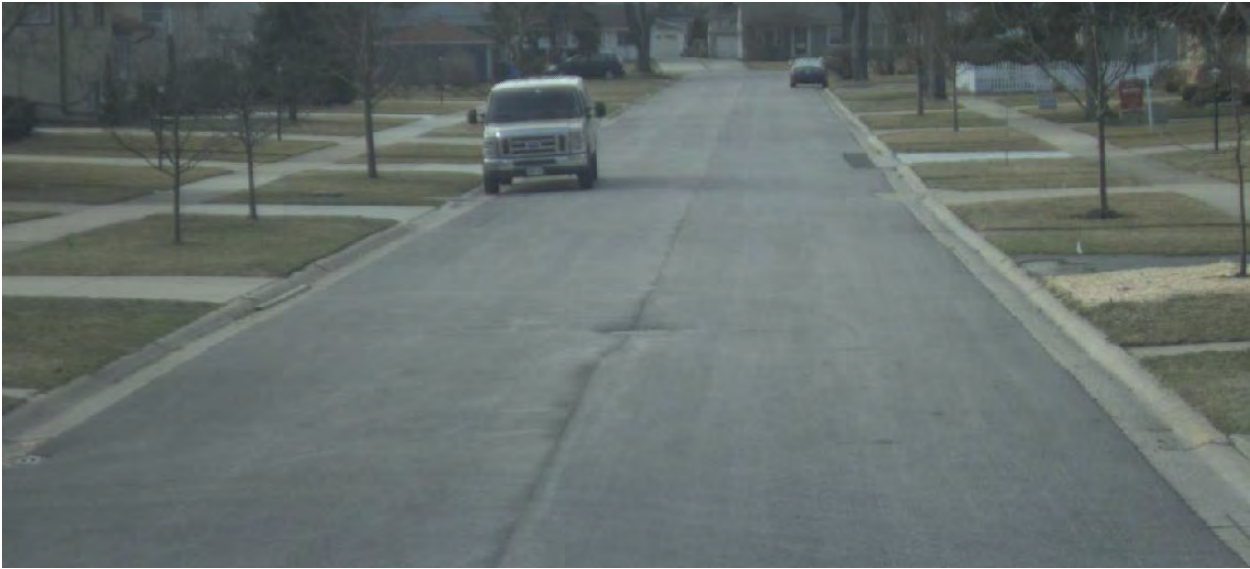
Figure 3-8: Locust Street Section 10, PCI 86 (Good)
