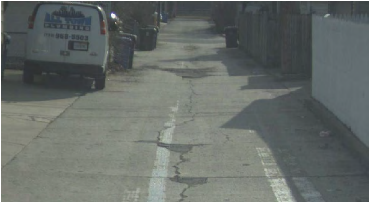
Figure 3-14: Oakton/Manheim Section A69, PCI 50 (Poor)
