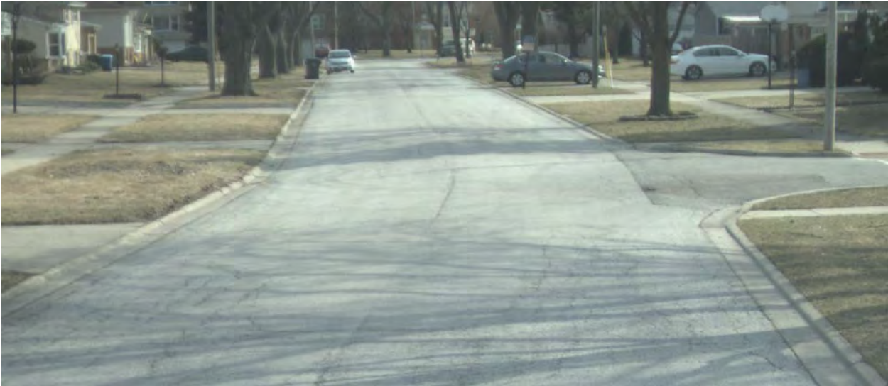
Figure 3-16: Hawthorne Terr Section 00, PCI 14 (Serious)
