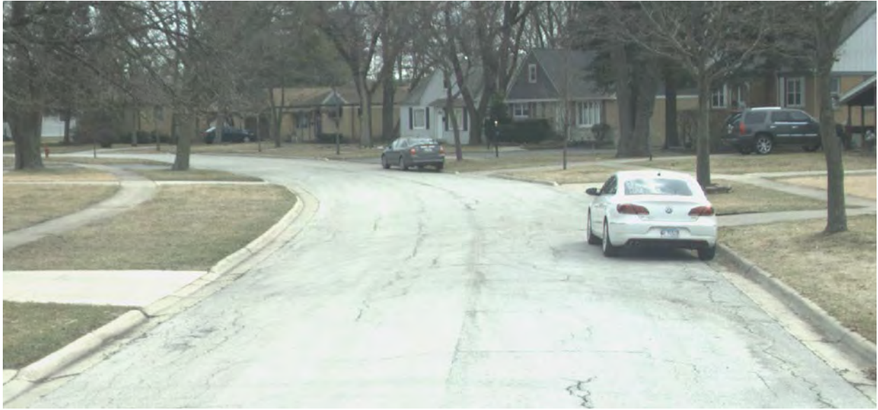
Figure 3-14: Oakton/Manheim Section A69, PCI 50 (Poor)
