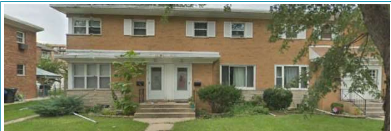
Figure 15. Typical building within Repetitive Loss Area 5. As shown above, many of the buildings in this area have extended their downspouts and sump pump discharges to drain away from the building.
