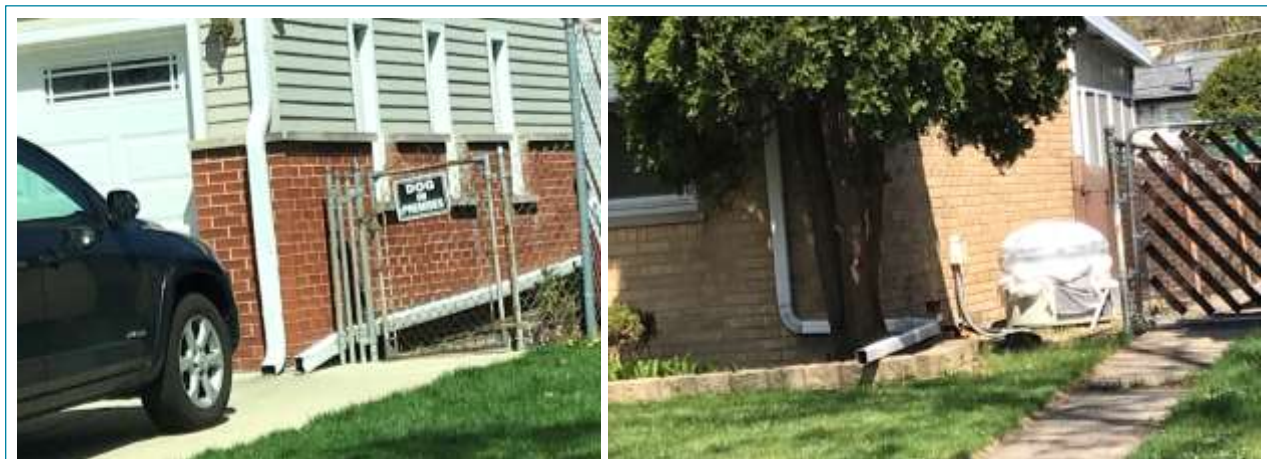
Figure 31. Typical Structures in Repetitive Loss Area 13. The property owners for both of the structures pictured above in Repetitive Loss Area 13 extended their downspouts to an area where the runoff would drain away from the structure.
