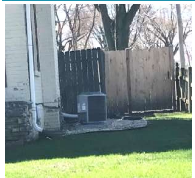
Figure 35. Typical Structure in Repetitive Loss Area 15. Structures in this area typically have at-grade air conditioning units and do not have extended downspouts.
