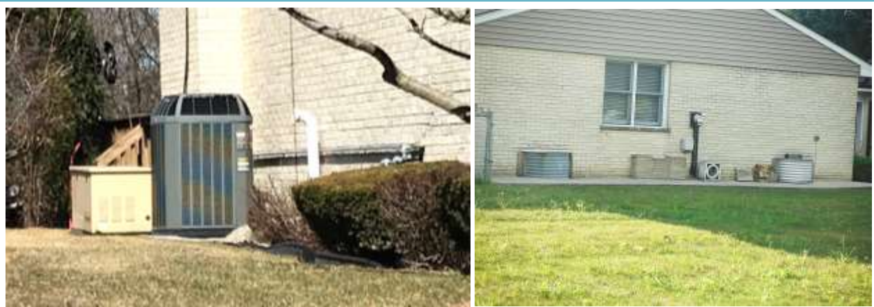
Figure 11. Generator and Raised Window Wells in RL 3. As shown above, residents in this area have generators and raised window wells to protect their homes from flooding.
