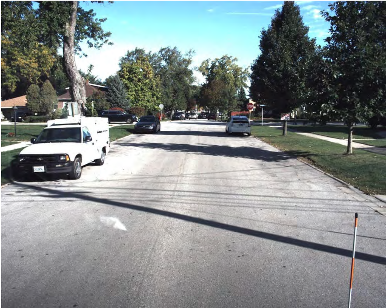
Figure 3-8: Ash Street Section 05, PCI 93 (Good)
