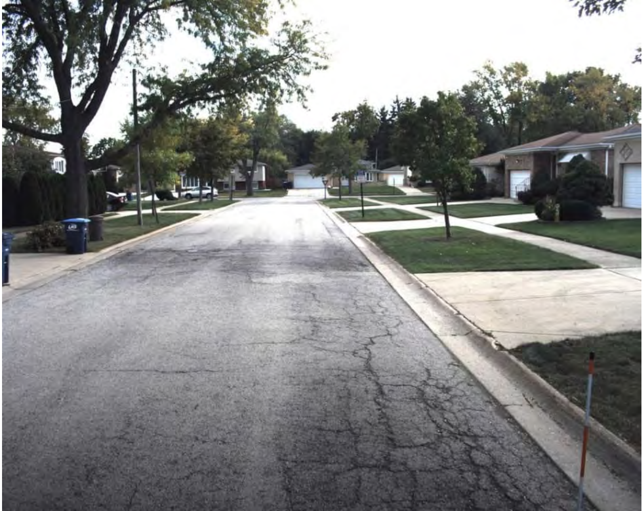
Figure 3-16: Joyce Dr Section 00, PCI 44 (Poor)
