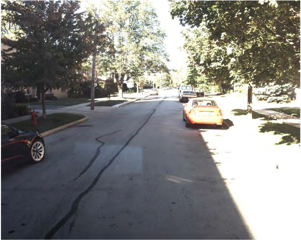
Figure 3-1: Alles Street Section 00, PCI 74 (Satisfactory)
