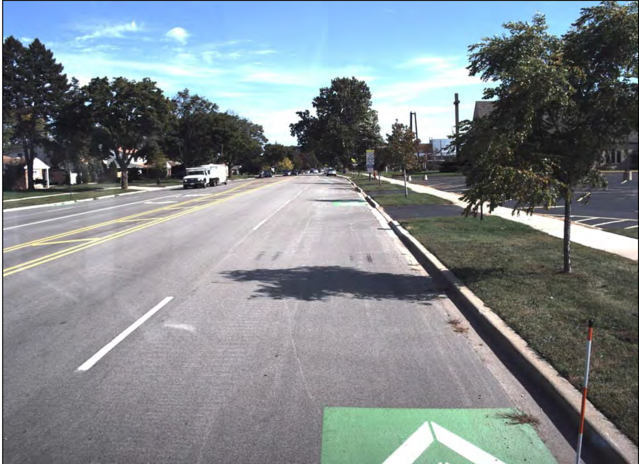
Figure 3-7: Algonquin Rd Section 05, PCI 95 (Good)
