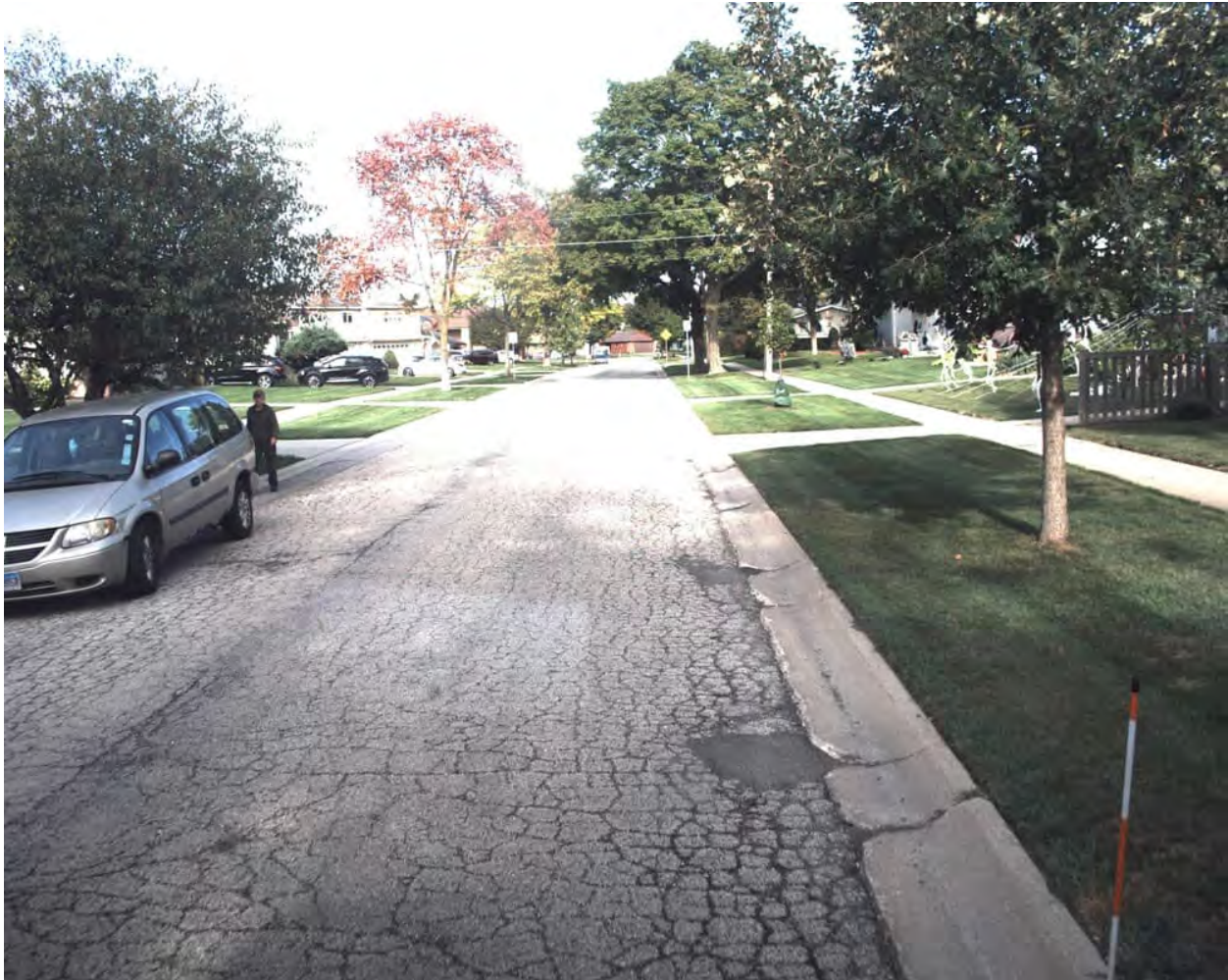
Figure 3-20: Waikiki Dr Section 00, PCI 13 (Serious)
