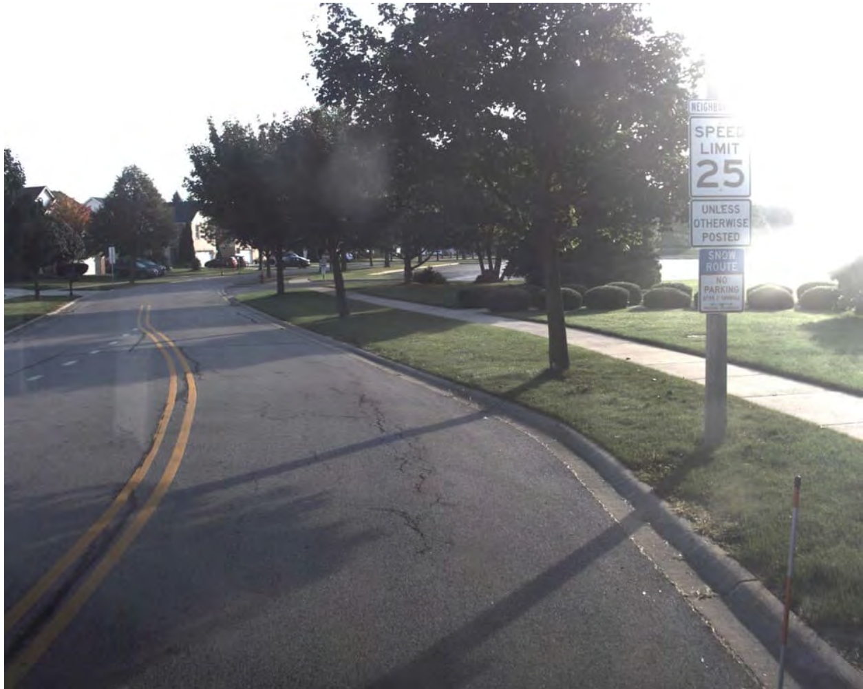
Figure 3-2: Dursey Ln Section 00, PCI 61 (Fair)
