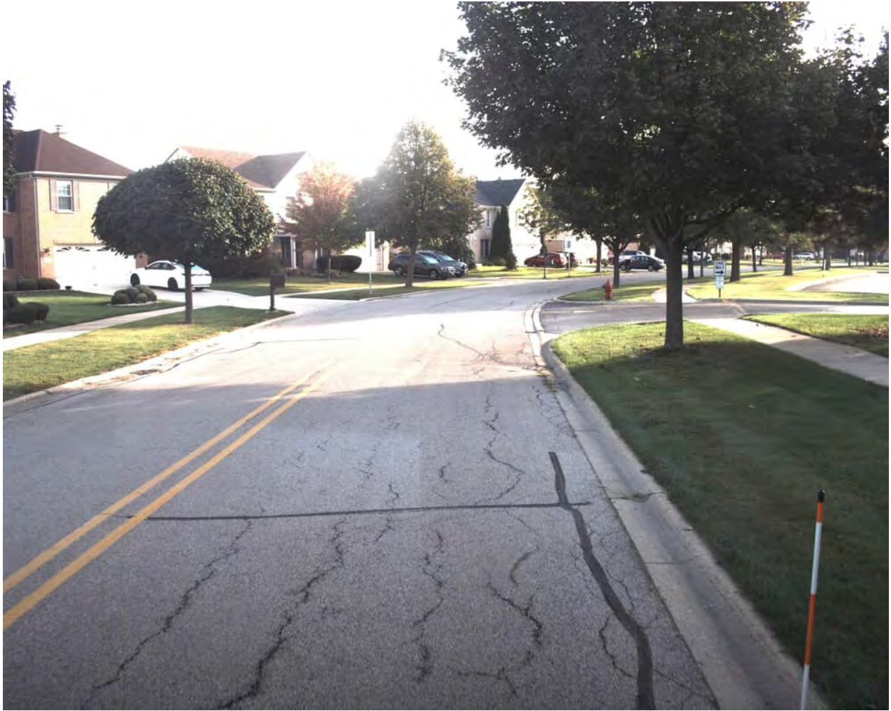
Figure 3-3: Dursey Ln Section 00, PCI 61 (Fair)
