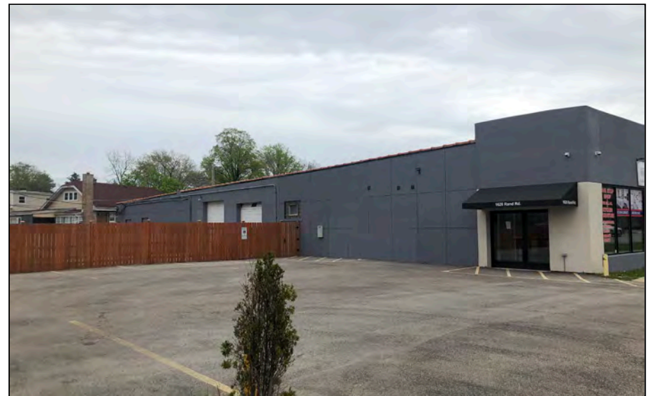
1628 Rand Road – Motor Vehicle Sales Entrance
