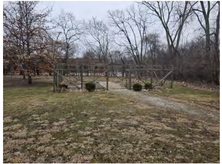
10. Southwest corner of existing building
