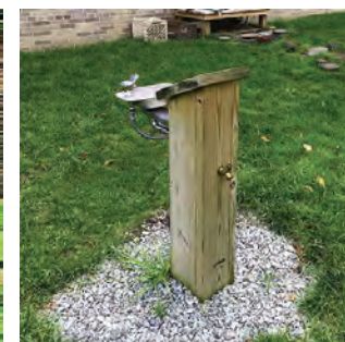
DRINKING FOUNTAIN WITH HOSE
