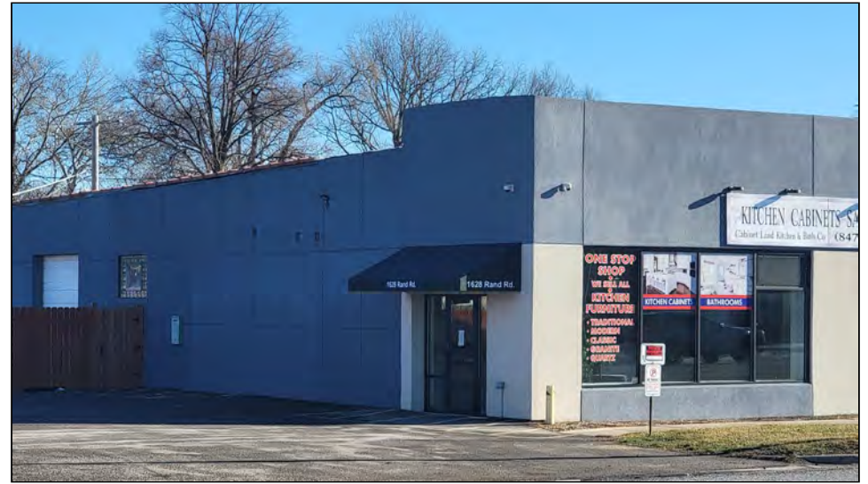
1628 Rand Road – Motor Vehicle Sales Entrance
