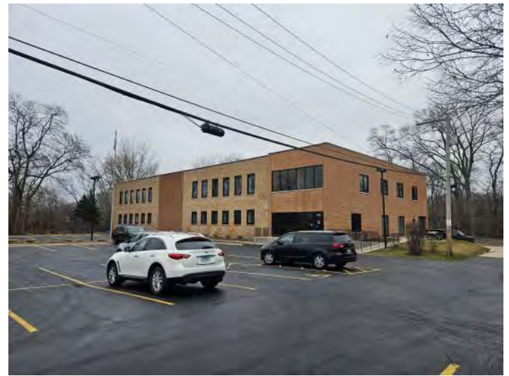
4. Southwest corner of existing building
