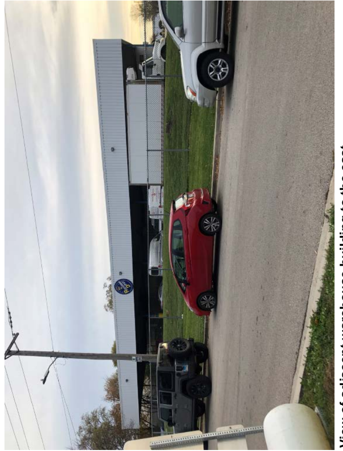
View of adjacent warehouse building to the east
