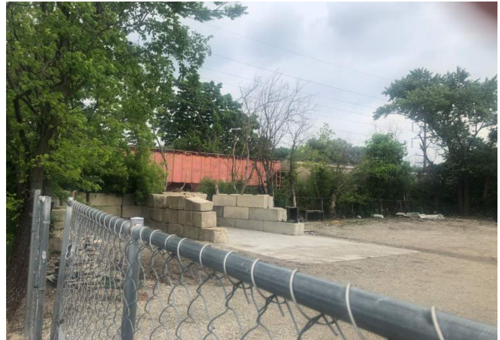
View of rear parking area with gravel, debris and dumpster enclosure.
