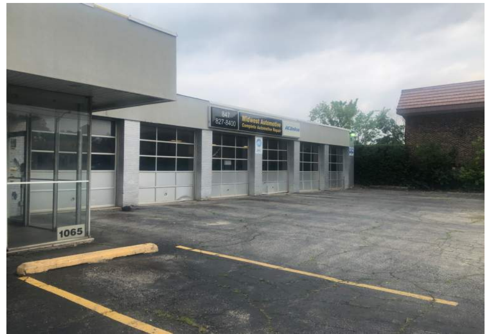
View of 6 work bays with overhead doors
