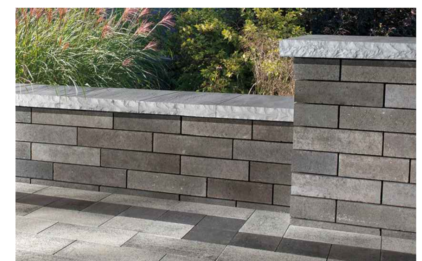
MASONRY SEAT WALL
