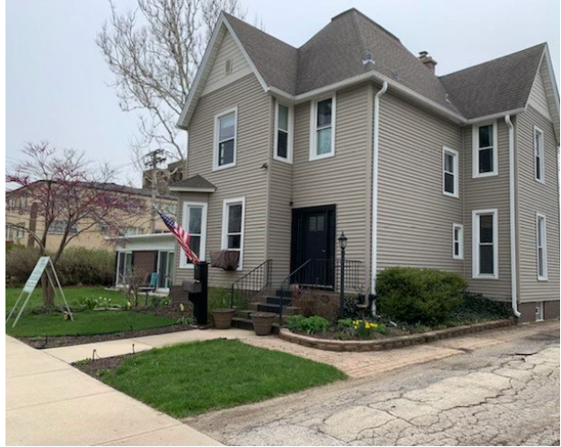
House, front (north) and side (west) elevations
