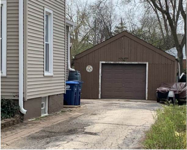
Existing detached garage
