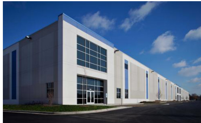
Northeast O’Hare Industrial Center.
