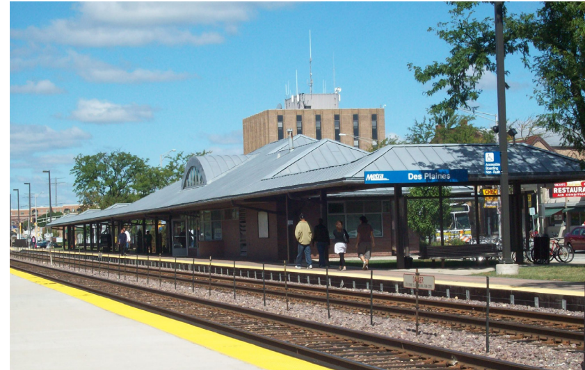
Des Plaines Metra Station. Photo credit: Strannik45
