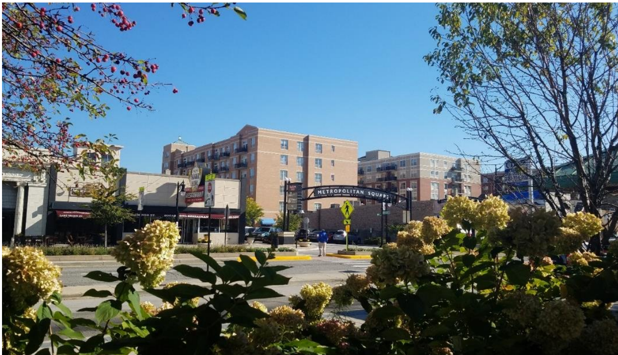
Caption: Metropolitan Square entrance on Miner Street in Downtown Des Plaines.
