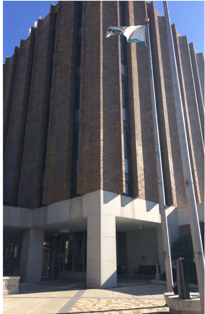
Des Plaines City Hall on Miner Street
