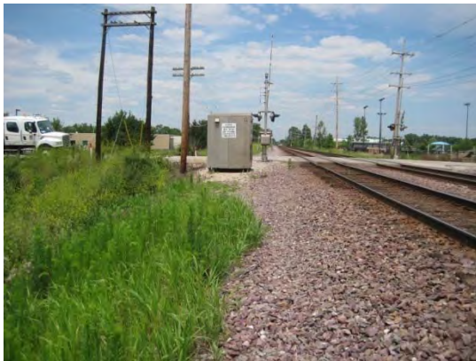
SIG BOX LOOKING NORTH
