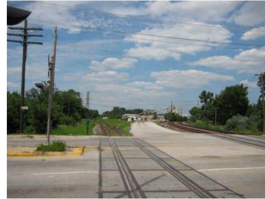
SPUR/UPRR LOOKING NORTH
