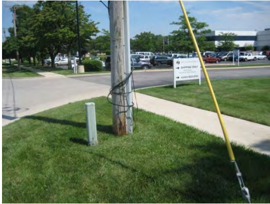
DRIVE LOOKING EAST
