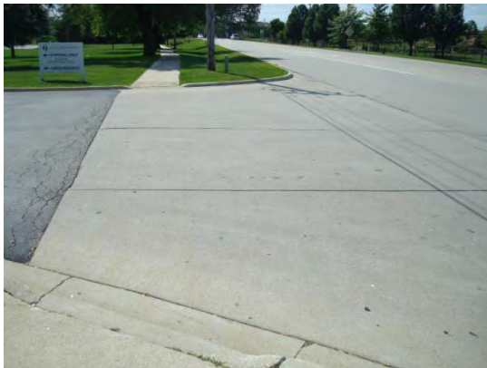
DRIVE LOOKING EAST
