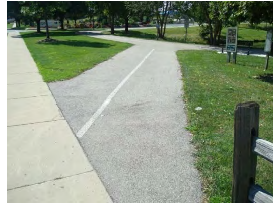
BIKE PATH LOOKING NORTHWEST
