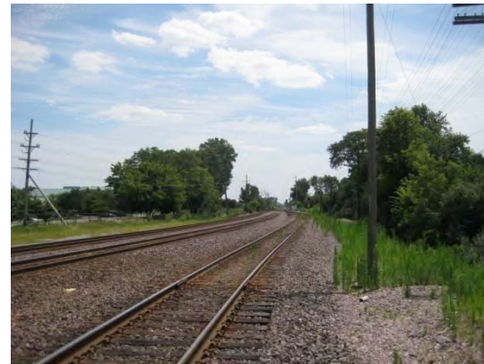
LEAD/UPRR LOOKING SOUTH
