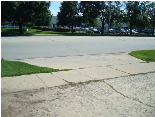
EAST DRIVE LOOKING SOUTHWEST
