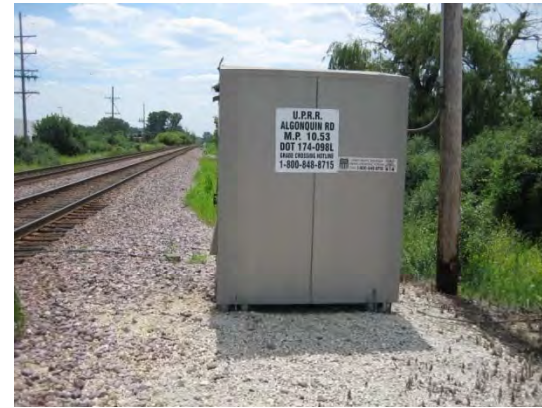
SIG BOX LOOKING SOUTH
