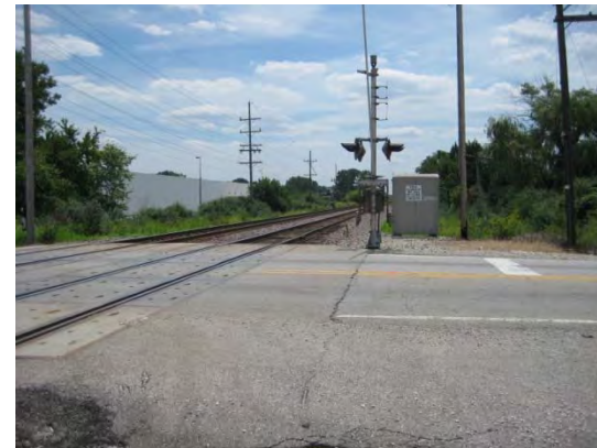
SIG BOX LOOKING SOUTH
