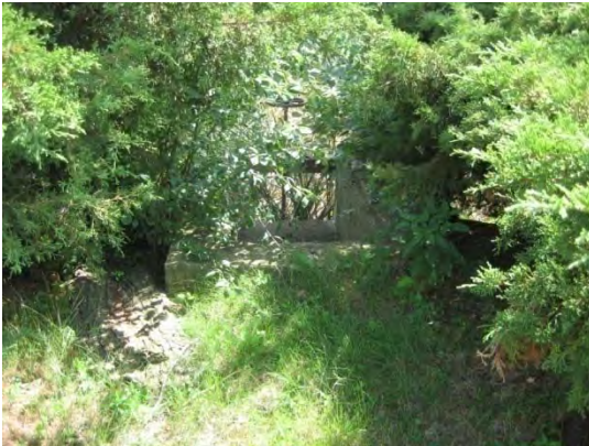
CONTROL STRUCTURE LOOKING SOUTH
