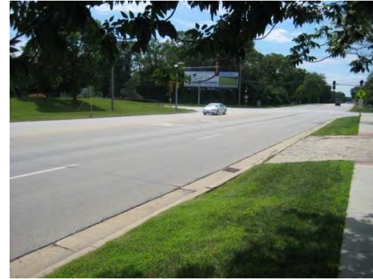
LOOKING WEST TOWARDS DRIVE
