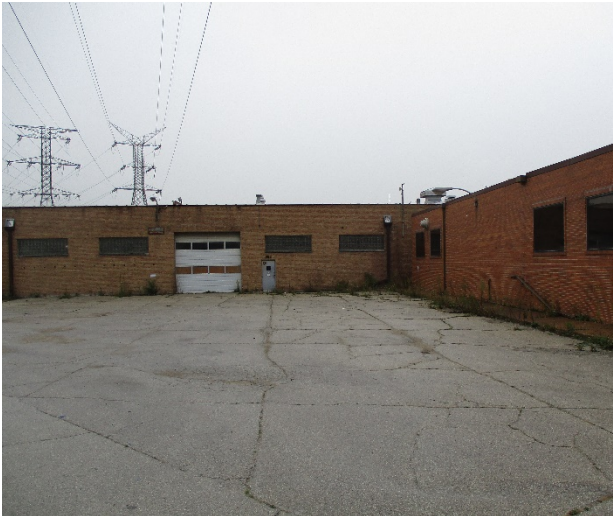
Existing building with overhead power lines
