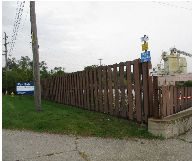
Existing fence at Wolf frontage/entrance with batch plant in background
