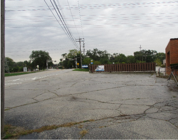
Looking south down Wolf Road at entrance
