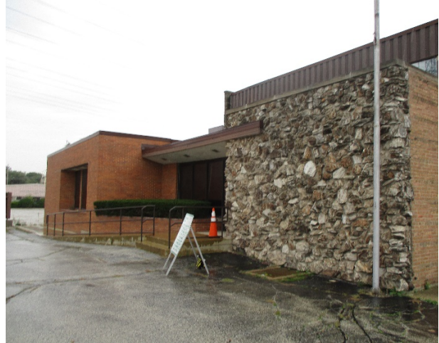
Front (east) facade of existing building
